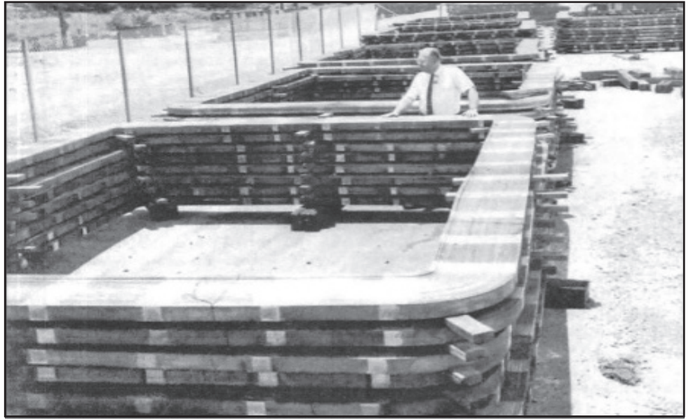
Silver-wound Magnet Coils for the Electromagnetic Process (Photo by Ed Westcott)
