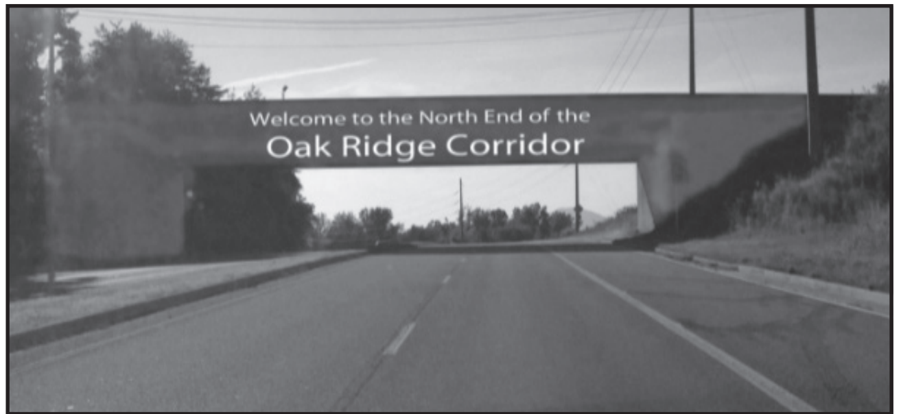
The bridge on Pine Ridge that crosses over South Illinois Ave would be an ideal location to recognize the Oak Ridge Corridor (Courtesy of Ray Smith)
