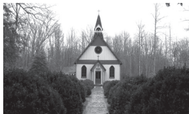
Across from the Rugby library is the Christ Church Episcopal chapel where the Rugby colonists worshipped in devotion to their "godly purpose." Provided by Historic Rugby
