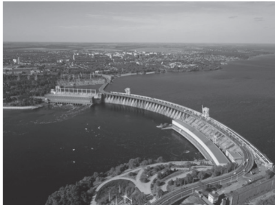
Zaporizhzhia-Dam, Ukraine Photo courtesy of Llya Pavlov
