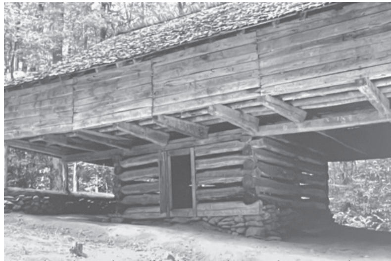
A cantilever barn. The small building on the ground supporting the cantilever barn section is the only part of the structure that is taxable.
