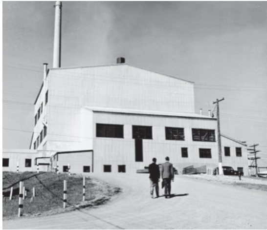
A view of the Graphite Reactor building from an unusual angle (Photo Submitted)
