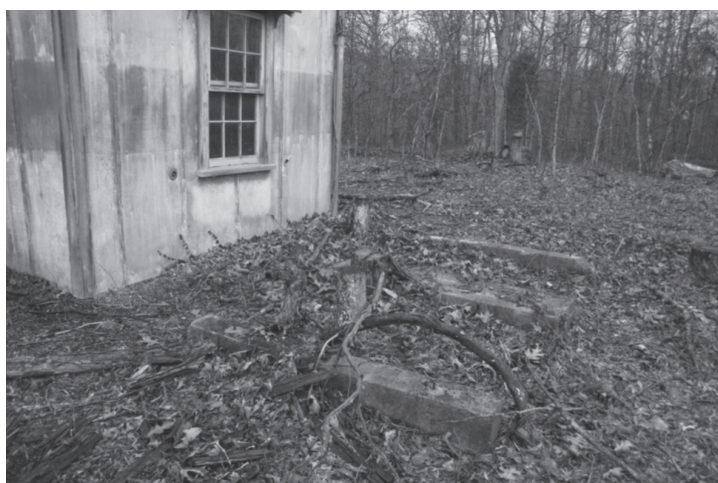
The two concrete foundations for the fuel tank obviously installed where the concrete arrow would have been had it been included in this installation (Photo Submitted)
