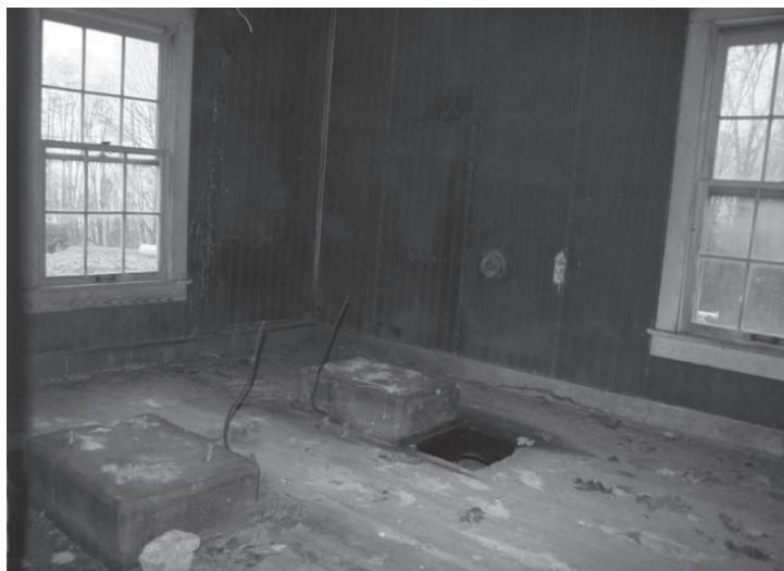
Interior of Beacon House showing concrete footers on which the generator sat that powered the airway light (Photo Submitted)
