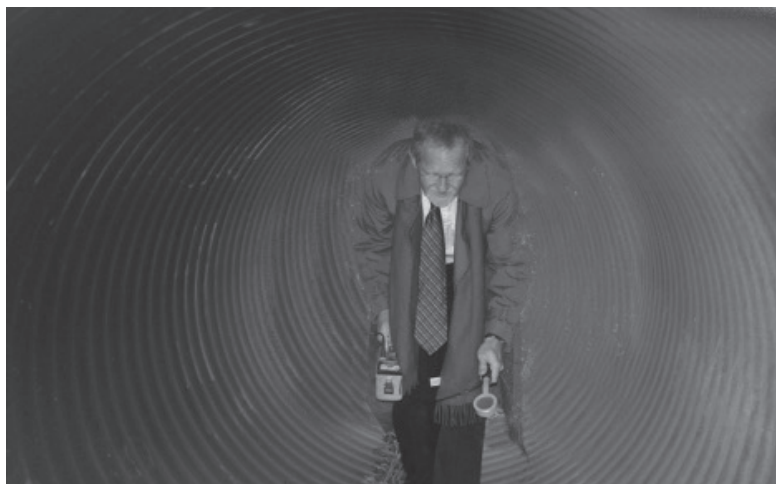
Jon Jefferson explored the storm sewer system in Oak Ridge. Here he poses in a large pipe to simulate the journey. Actually, he was much more appropriately dressed and did NOT have a Geiger counter! (Photo Submitted)
