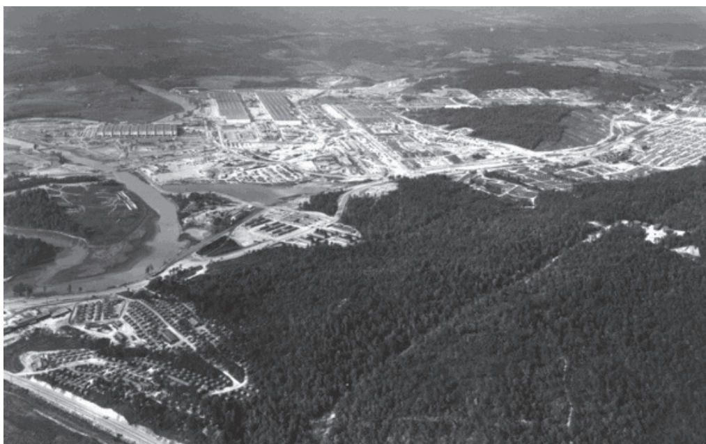
Sprawling Happy Valley and other construction camps near K-25 are shown all around the construction site in this aerial photograph of the Manhattan Project K-25 site (Photo Submitted)
