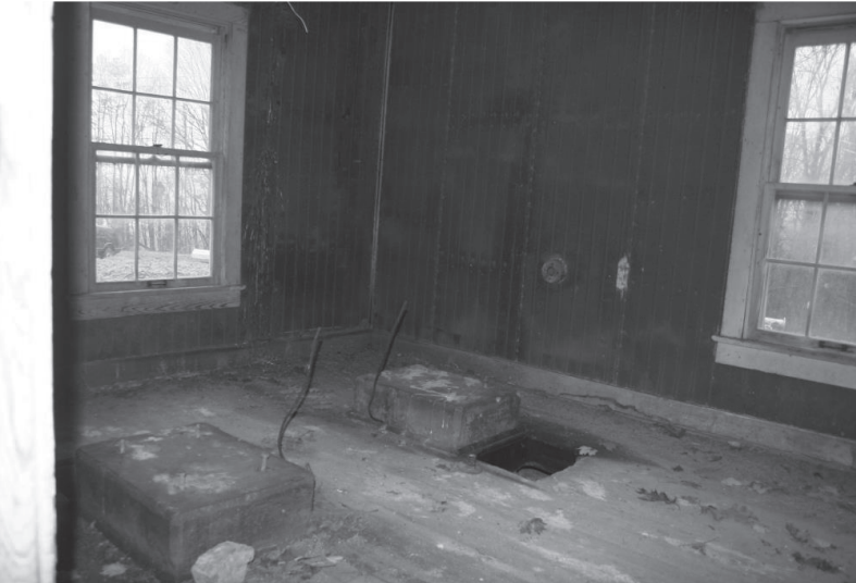
Our Beacon House located near the Oak Ridge National Laboratory The location where the generator would have set on the two concreted foundations. (Photo Submitted)
