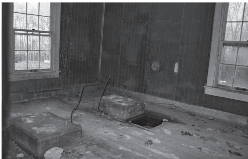
Interior of Beacon House showing concrete footers on which the generator sat that powered the airway light (Photo Submitted)
